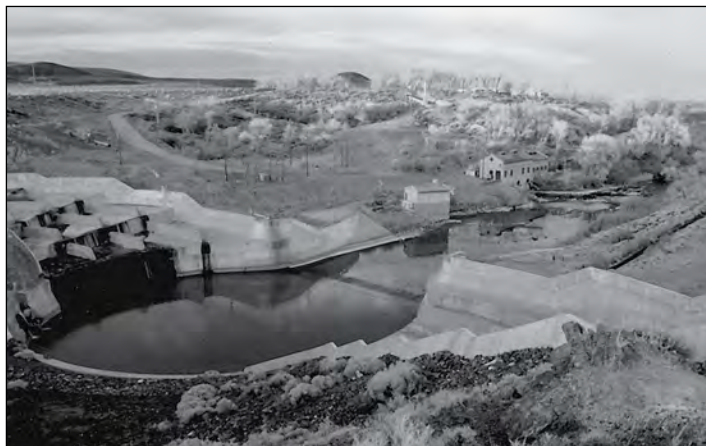
Lahontan Dam spillways and powerhouse on the Carson River Author's photo, 1993
